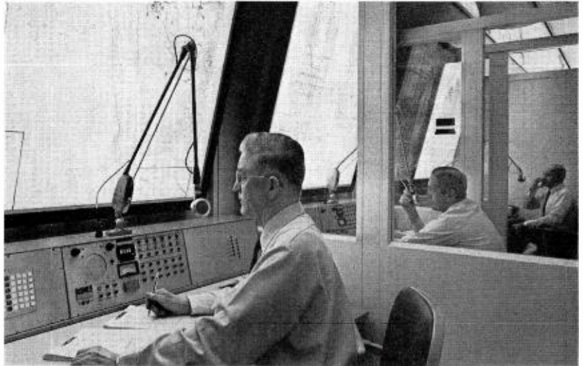
Three of 19 consoles in net's big control center where backlighted maps show radio dispatcher the bus routes he covers.
