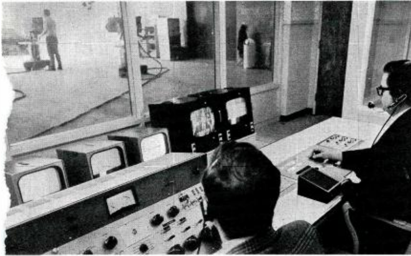
FIG. 16 Each studio has its own control room as shown above, containing the BC-8 audio console, PTS-1 switching system, remote controls for VTRs and film chains.
