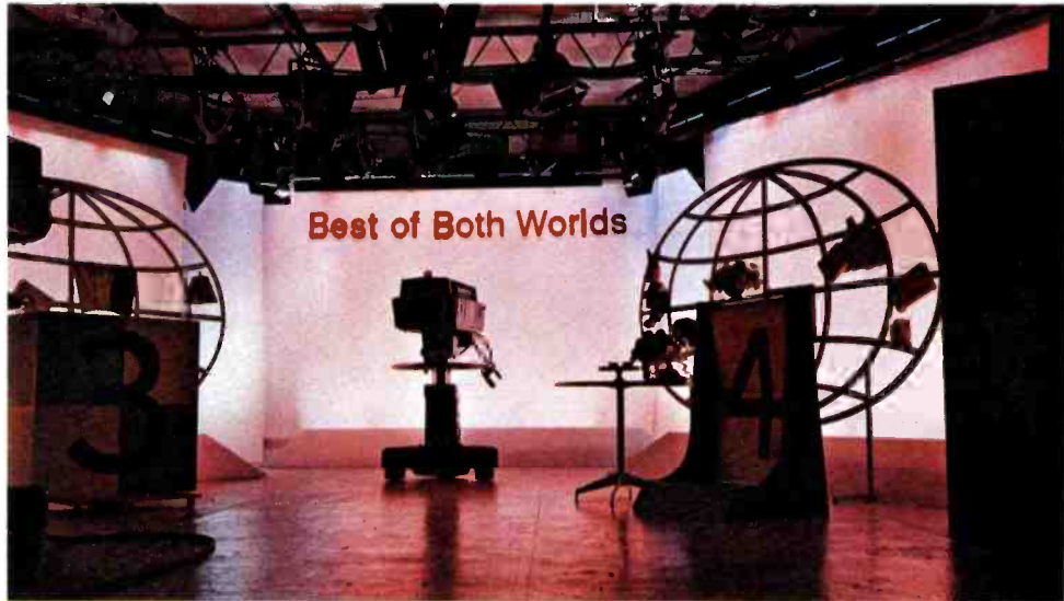
CYC AND SCRIM enclosed the color demonstration studio. Striplights, overhead and floor, used new plastic gels, in the primary colors, to produce a wide variety of color backgrounds. Quartz fixtures, supplied by Colortran, were used throughout the studio. The basic simplicity of the set demonstrated the kind of sophistication color lighting can bring to color TV pictures.
